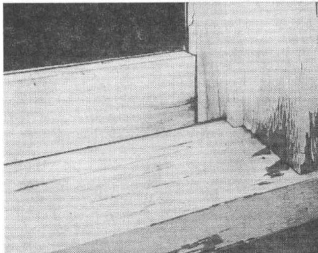
**Figure 2. Effect of water repellent preservative (WRP) on service life of window unit: (top) window unit pretreated with WRP prior to painting; (bottom) untreated window unit. Paint degradation caused by water absorption into end grain.**
