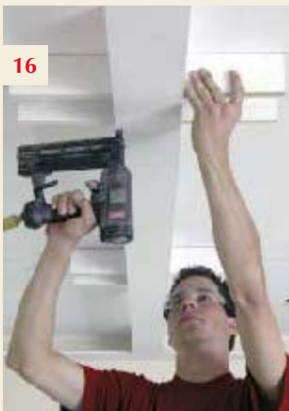
**16.** Fasten the soffit to each piece of backing, but just tack it with brads so it will be easier to string the beam bottoms straight.
