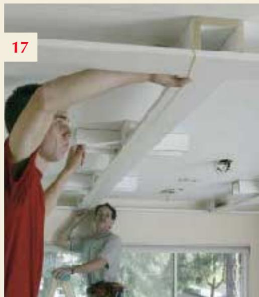
**17.** On this job, we didn't have to make the beams perfectly straight. This built-up cornice has large reveals between each piece of molding, which hides a lot of sin in the ceiling. Using a string and some long shims, we just got them close to the eye — within 3/8 inch. But with some designs, the beams must be installed almost perfectly straight.
