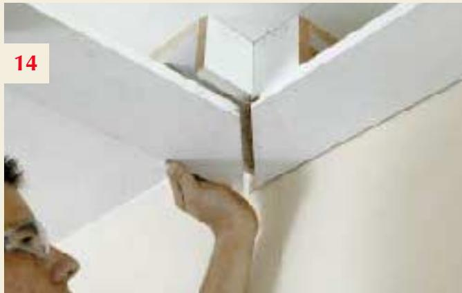
**14.** We cut splines from 1/4-inch MDF because it's exactly the right thickness. Glue the kerf on the installed piece and insert the spline, then apply a liberal amount of glue to all surfaces of the spline and to the shoulders of the miter before installing the second board.
