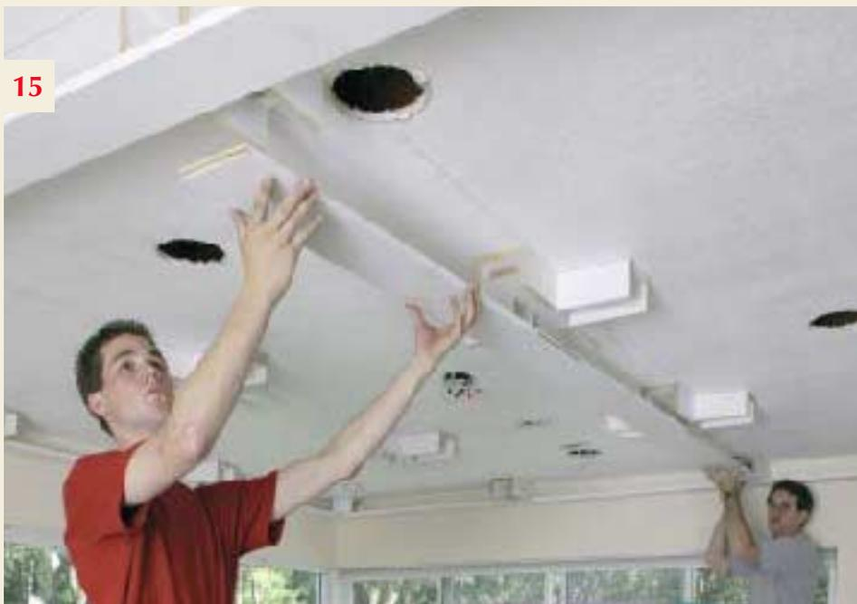
**15.** Install the center beam bottoms next, splining those butt joints to the perimeter soffit. Cut all the pieces a hair long and spring them into place. Run the kerfs long so splines can be slid into place after the pieces are in position. Remember, the long kerfs will be covered by the beam sides.
