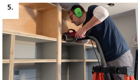
5. Cut corresponding slots on cabinet boxes
