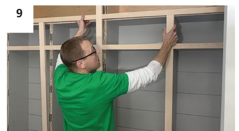
9. Install face frame
