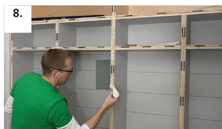
8. Apply glue (when using Tenso)
