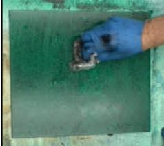
Dab the rag onto the glaze. Rewet with Mineral Spirits as necessary.
